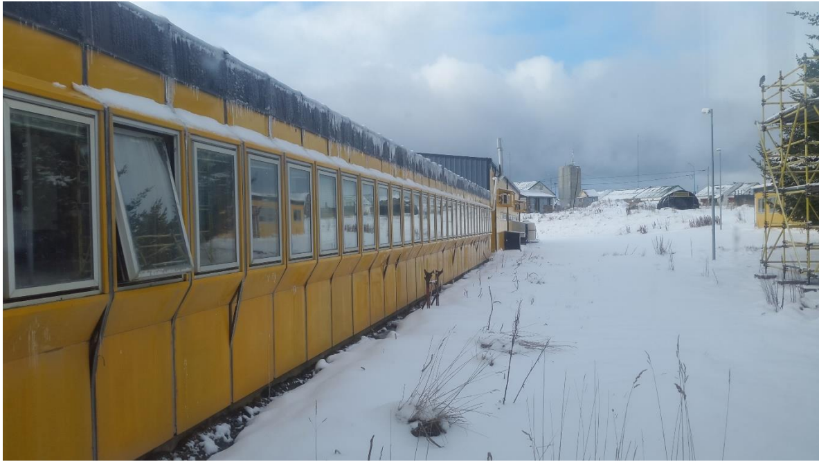
Figure 5.1. Picture of the installations of CADIC connecting offices and houses (2019)
